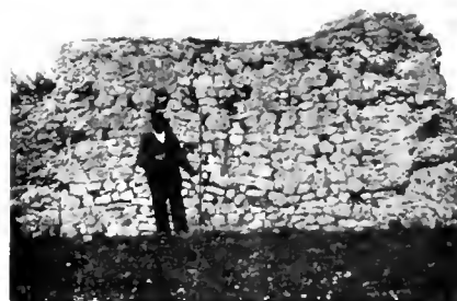
4 A PIECE OF THE MURO PERTUSO BETWEEN THE View from the south
